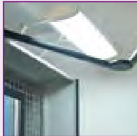
Lighting of the space between units. The illumination is controlled electronically and works only above the unit currently used by personnel. Lighting covers are placed on metal trusses, screwed to the top shelves (the covering). The illumination starts automatically when the alley is opening and switches off when it is closing, provided software allows user to set the time after which the light is switched off.
